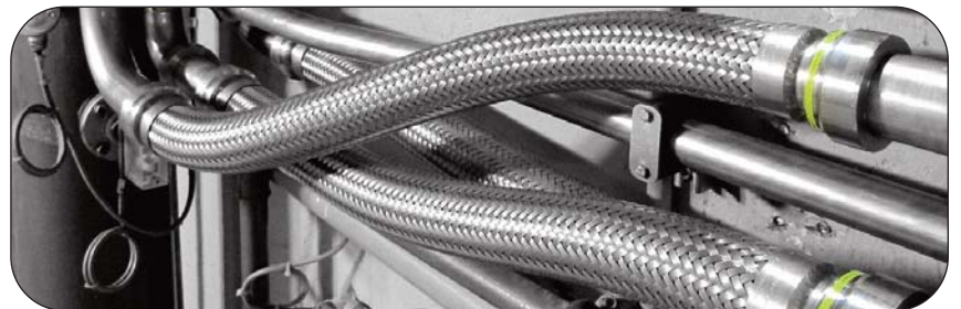
Thorburn Model NS96Z installed in a nuclear power plant
