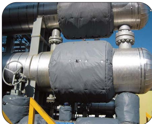
Thorburn's ThermaCover™ can be used for freeze protection and heat retention
