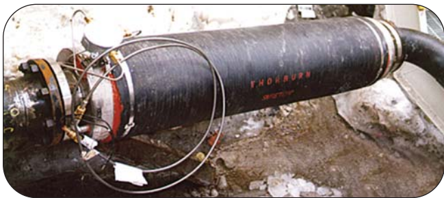
Thorburn's Sure-Temp hose assembly transporting bitumen
