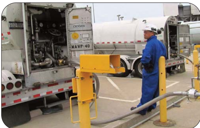
Compressed Gas Bulk Loading Station
