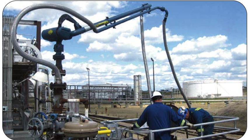
Thorburn’s (N)M95 Monel hose assembly attached to a rail loading arm
